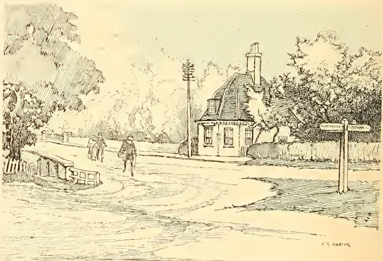
OLD TOLL-HOUSE, STRATFORD BRIDGE.
